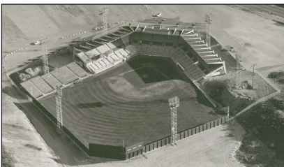
Aerial view of the newly-completed Cheney Stadium - nicknamed the "The 100-Day Wonder" due to its brisk construction schedule.
