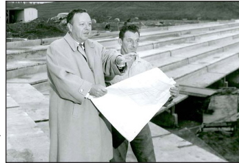
Ben Cheney surveying the early stages of the stadium prior to the Tacoma Giants first season in 1960.
